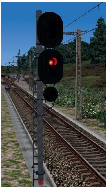
RED: It is forbidden to pass this signal – the points are not set, or there is a train ahead.
